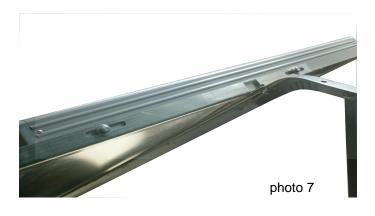
Secure the collectors on the frame using the bolts,
